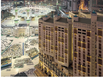
Millennium Hotel Makkah, KSA
