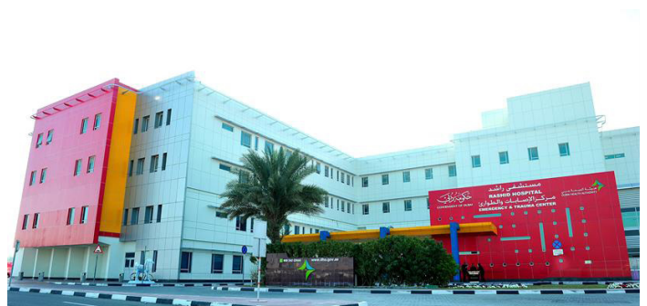
Rashid Hospital Expansion, Dubai, UAE
