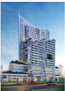
Al Shirawi Commercial Building Business Bay, Dubai, UAE
