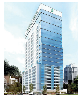
Dubai Islamic Bank, Headquarter, Dubai, UAE
